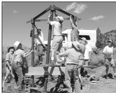
The crew lifts the header beam onto the posts for the Heenan Lake display.
